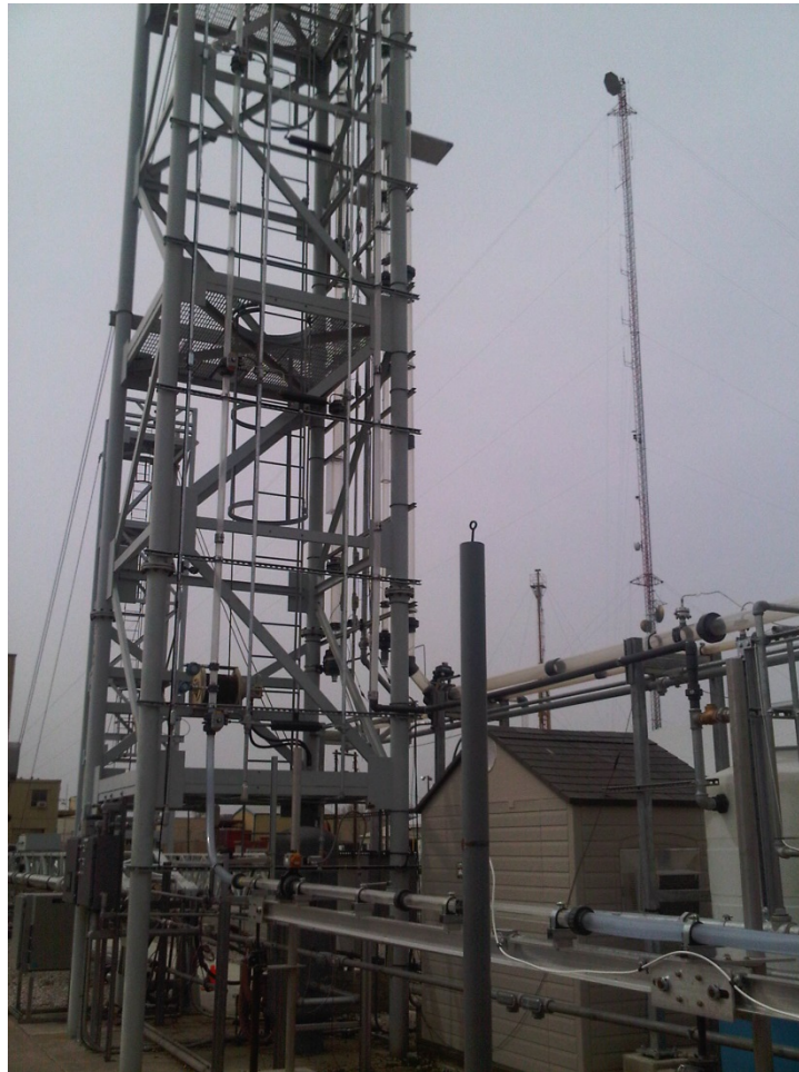
Figure 6. 2-in. Horizontal Well Experimental Facility
