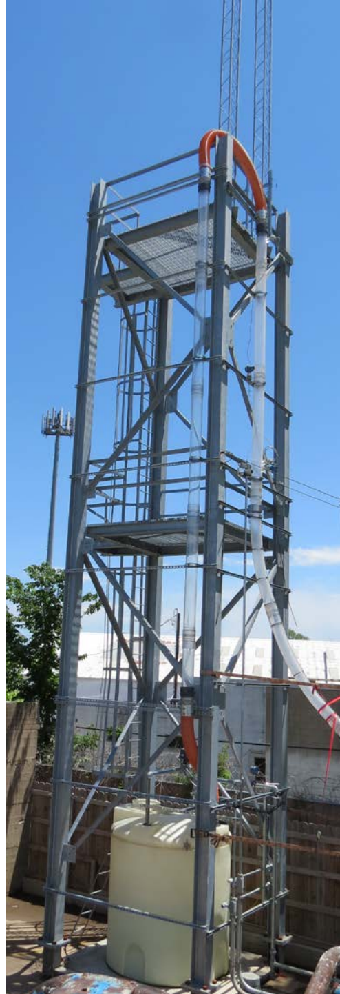
Figure 5. Tower of 6-in. Horizontal Well Facility
